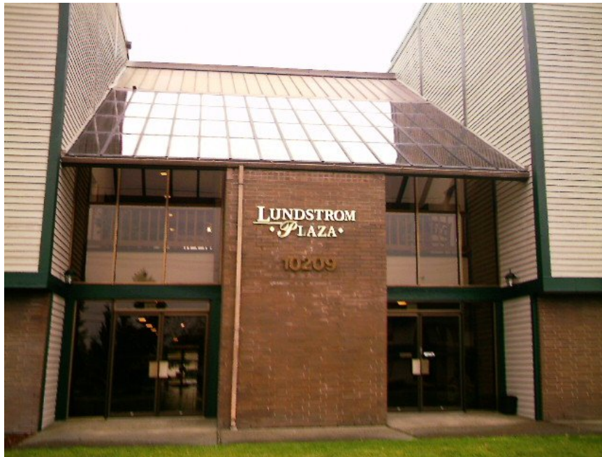
The front view of our building as you drive past it on Bridgeport Way SW. The Seminary and Church Ministries are located on the main floor.
